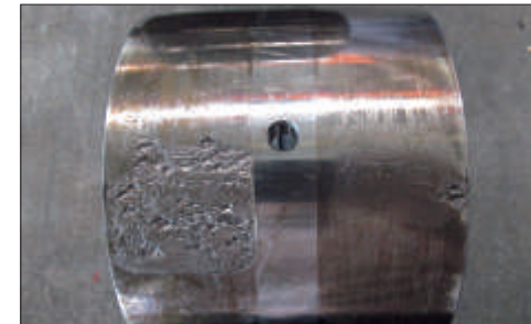
Photo 1-13 Part: Inner ring of a cylindrical roller bearing for sendzimir Mills Symptom: Flaking occurs on the raceway surface Cause: Severe operating conditions and oil lubrication of low viscosity
